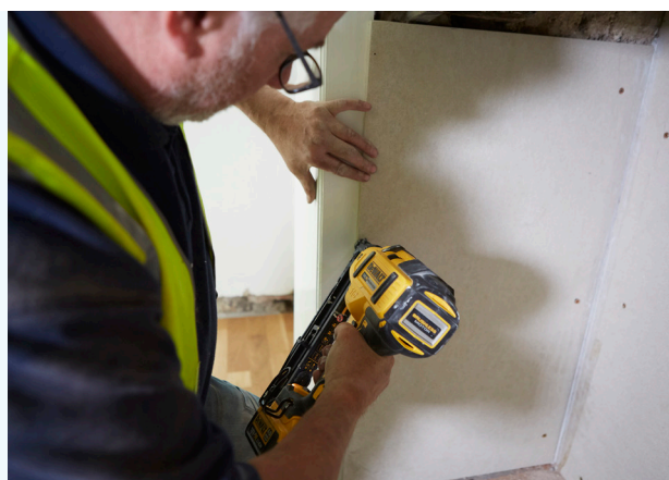
Fixing using a nail gun.
