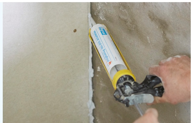
Applying PROMAFOUR® Glue to the back left and right corners.
