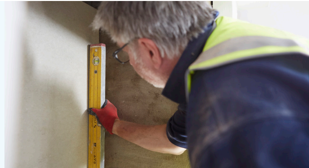
Checking the board is level.
