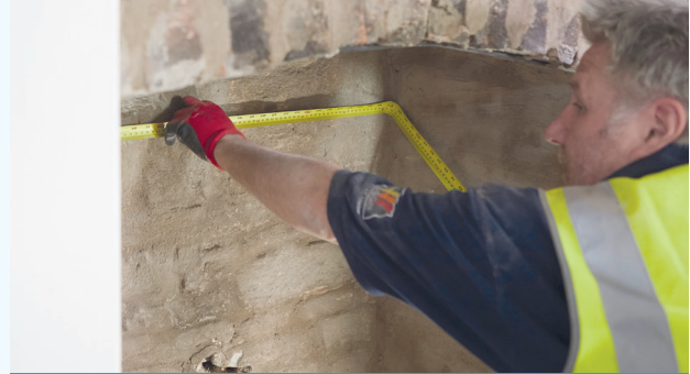
Measuring the surfaces of the fireplace.
