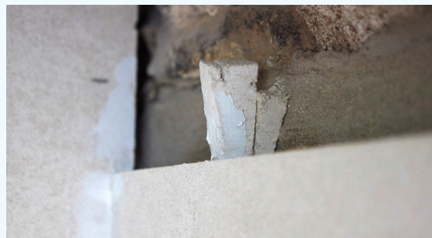
Using a PROMAFOUR® wedge to correct uneven walls.
