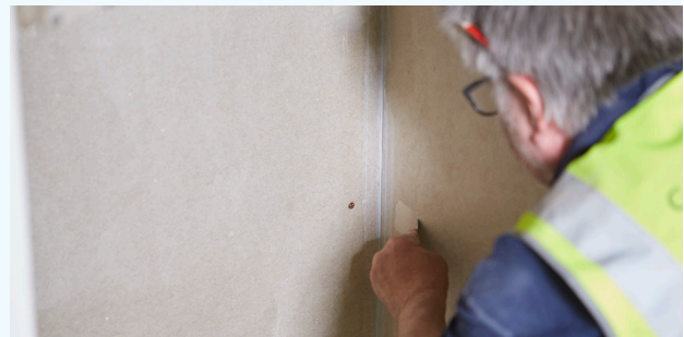
Once dry PROMAFOUR®-HT Joint Filler can be sanded down.
