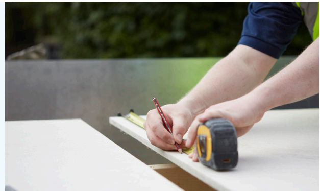
Place your measurements on the board prior to cutting.
