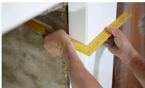
Using a right angle set square to check for uneven surfaces
