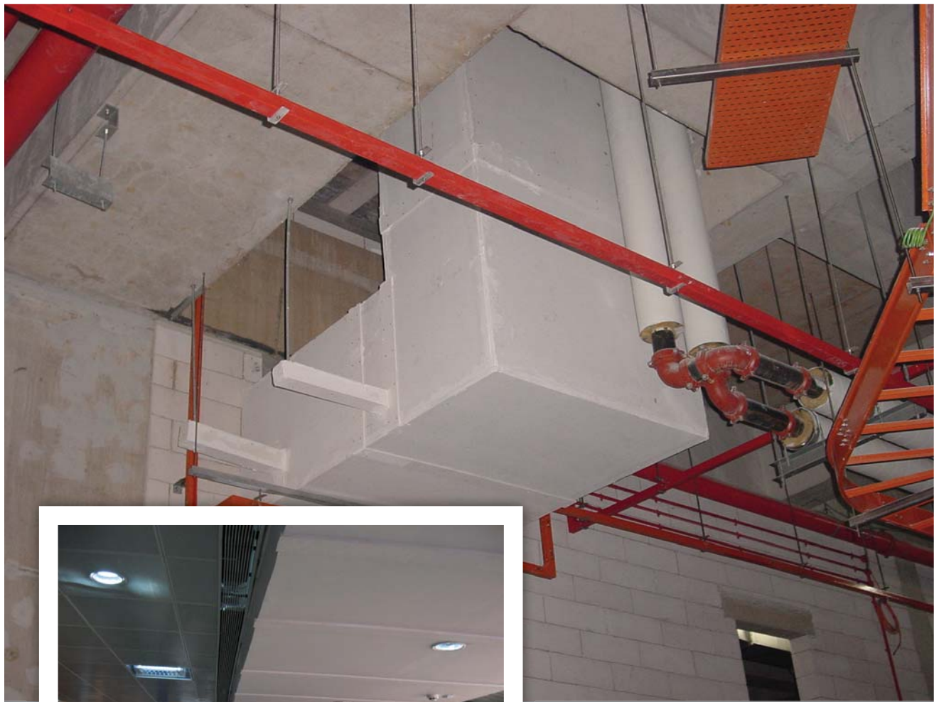
Steel duct claddings inside the Changi Water Reclamation Plant (above) and the boarding hall of Pune International Airport in Maharashtra, India (left). Both projects used PROMATECT®-H boards.
