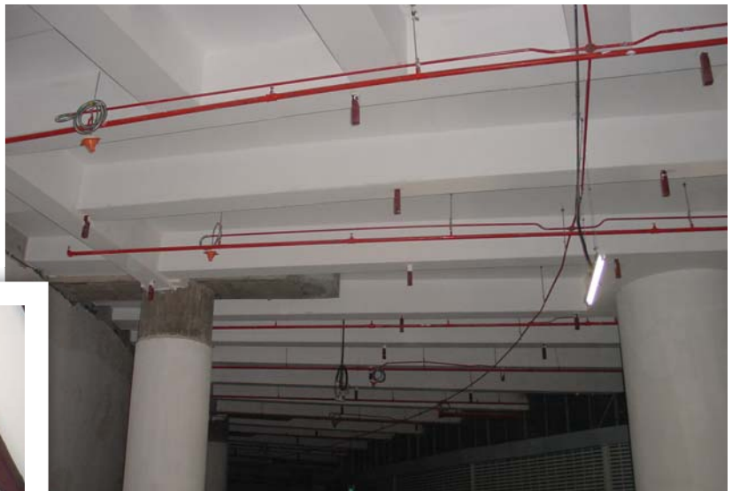
Above PROMATECT®-H self-supporting ceiling membrane, at time of construction of Terminal 3, Changi International Airport, Singapore.
