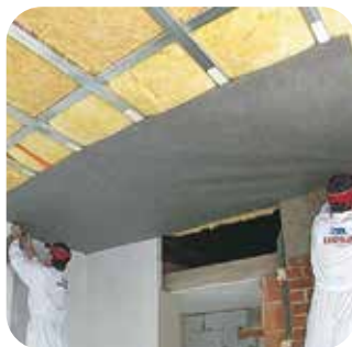
4. Namestimo parne ovire URSA SECO PRO 2 ( s_d \approx 2 \text{ m} ) ali parne zapore URSA SECO PRO 100 ( s_d \geq 100 \text{ m} )
