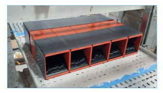
EZ Path<sup>®</sup> installed inside the cable tray and centered inside the wall.
