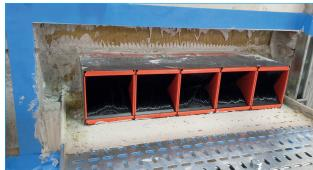
EZ Path® installed inside the cable tray and centered inside the wall.
