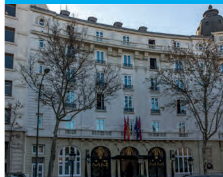
REFORMA HOTEL RITZ (MADRID)
