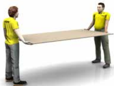
Figure 2 Whenever possible, lift the panel from the stack below rather than slide panel or drag off the stack. This will prevent damage by scratches to the lower panel.
