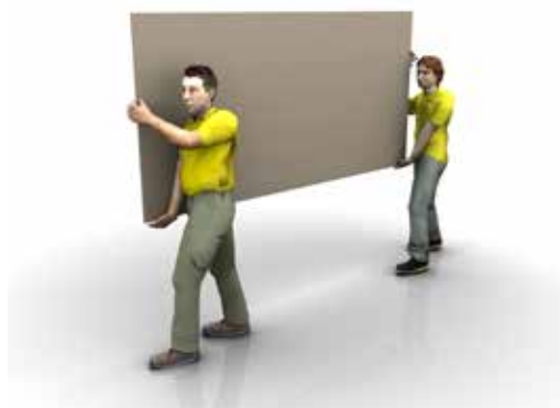
Figure 3 Always carry the panel on edge but DO NOT store on edge
