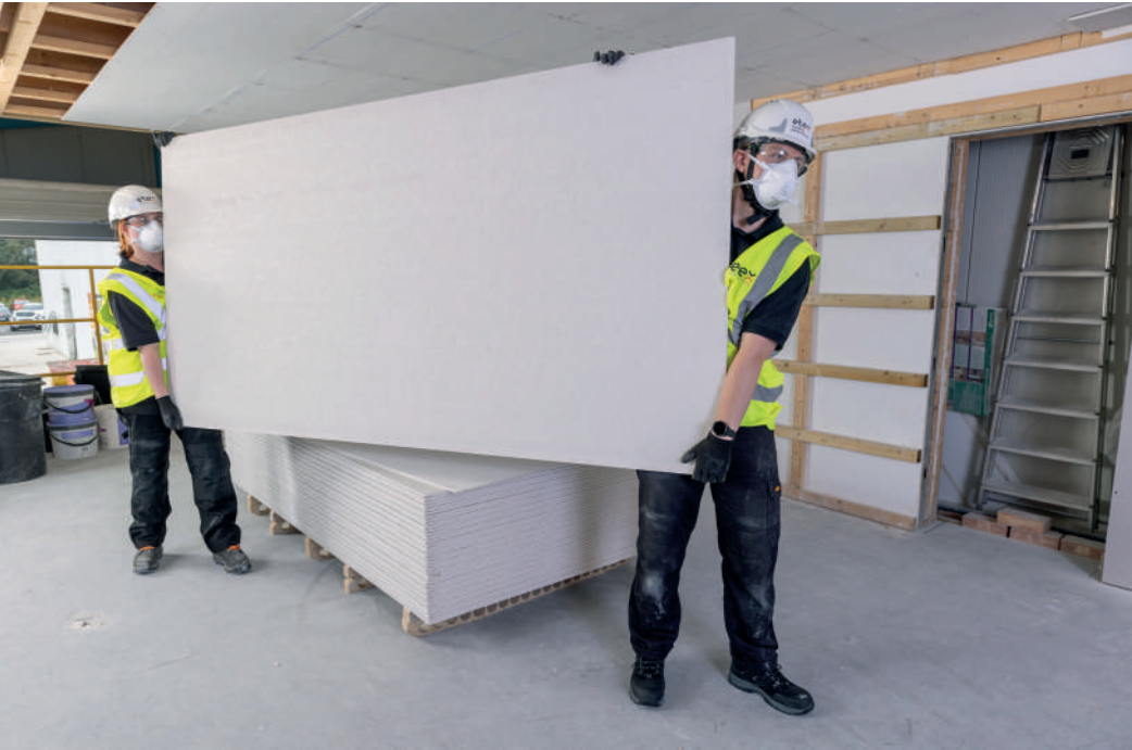
b) Always carry the boards on edge but do not store on the edge.
