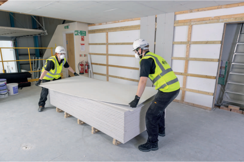
a) Wherever possible, always lift the boards from the underside rather than sliding the boards on each other on the stack, to prevent damage or scratches on surface of the boards.
