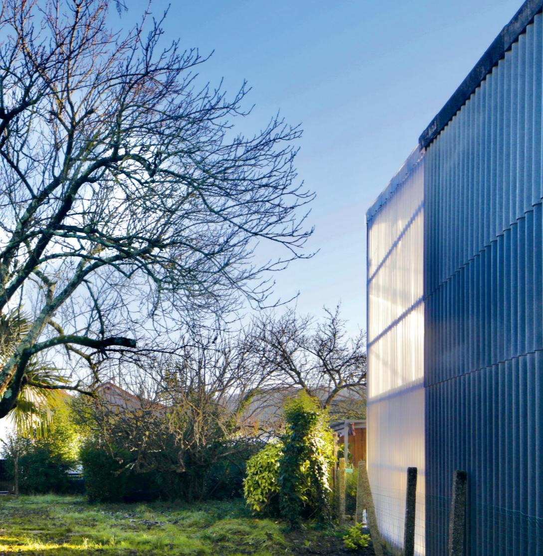
When closed a continuous, seemingly impenetrable facade of corrugated fibre cement sheets is created. Special eaves elements enable the corrugations to be continued directly into the roof cladding and the gutter can be inserted in the roof so that it is not visible from outside.
