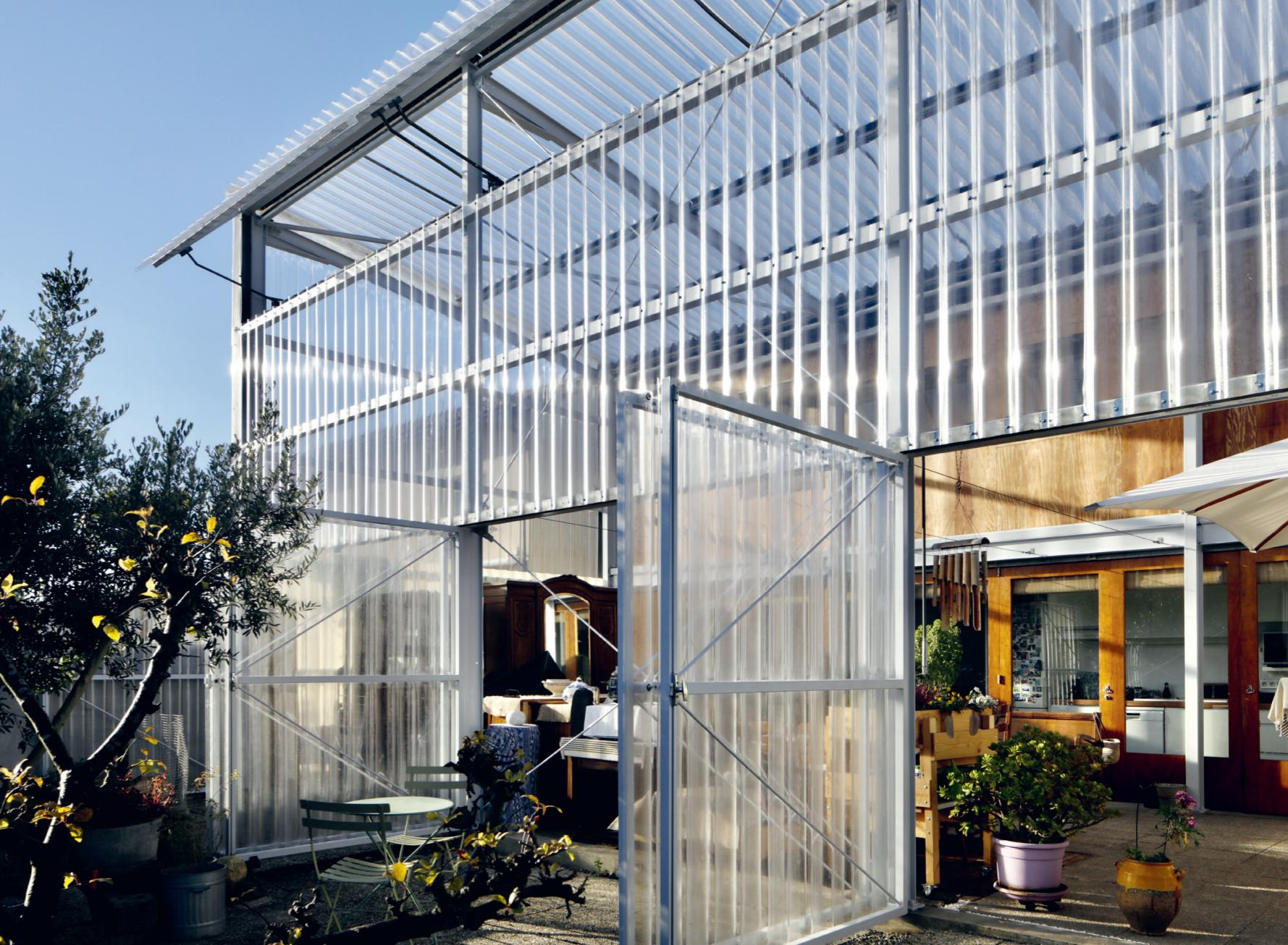
The bedrooms and living rooms are on two floors. A central space-saving stairs provides access to the upper level. On the ground floor the large steel doors clad with corrugated fibre cement sheets can be opened completely, on the upper floor the opening elements can be tilted upwards to reveal the view.
