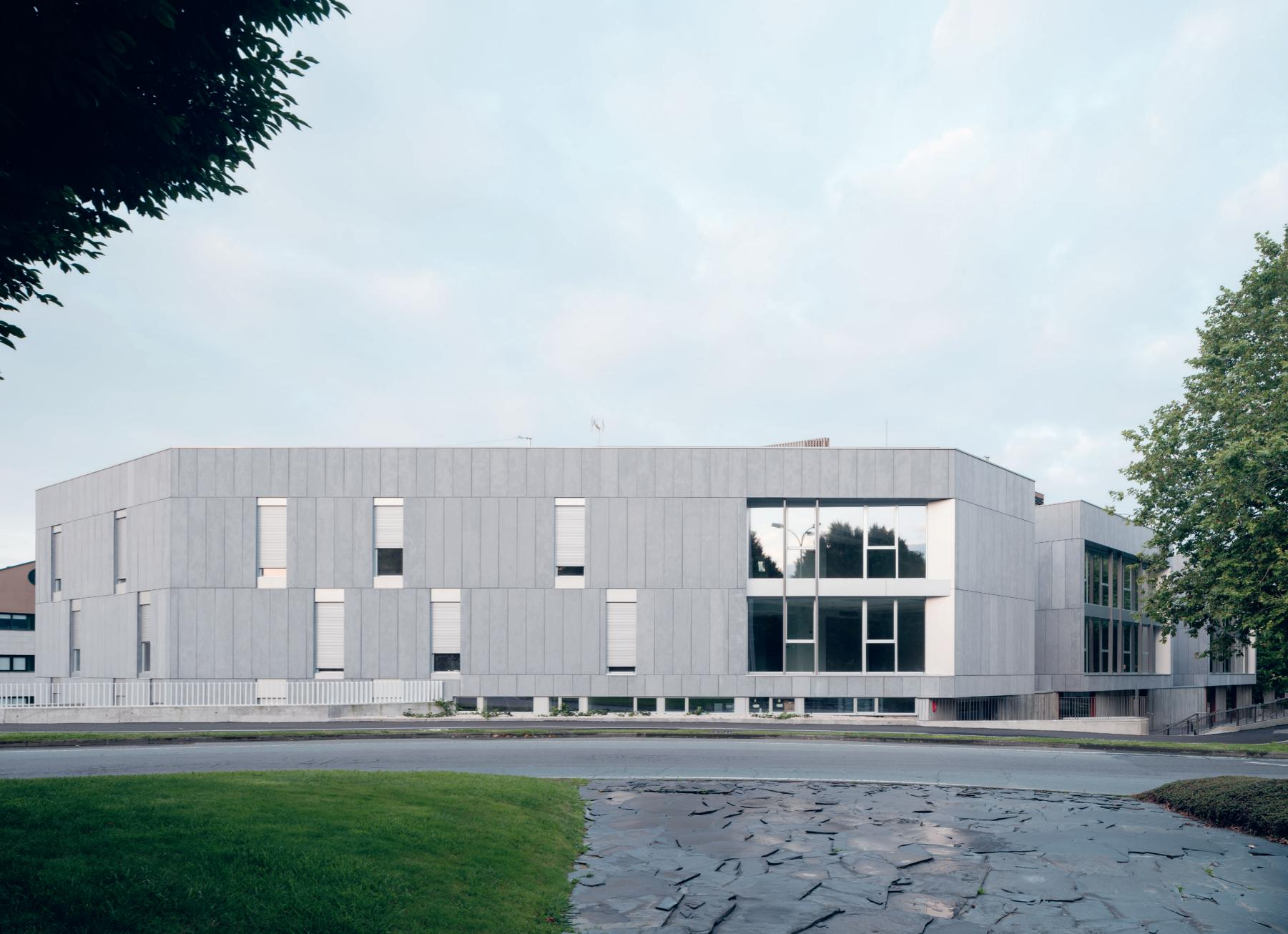
Through their fine surface structure, the light grey fibre cement panels are a strong contrast to the rough untreated reinforced concrete, which is the structural and design basis for the building as a whole.
