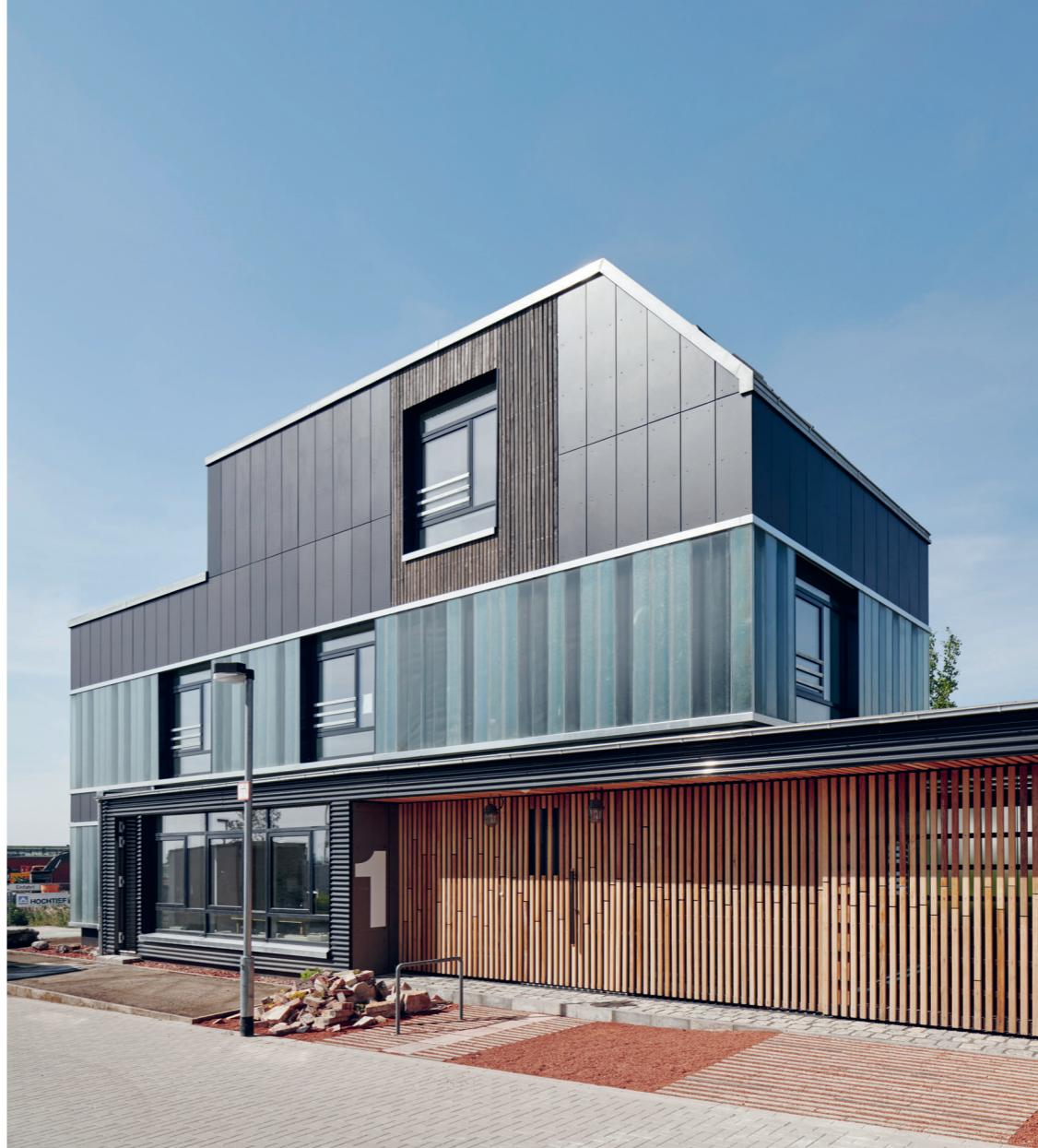
The simple rectangular plan of the narrow building is continued on all three levels. On the top floor a roof terrace was cut out of the volume. The transition between the black-coated fibre cement panels and the profiled glass elements was made using metal sections that are clearly visible.
