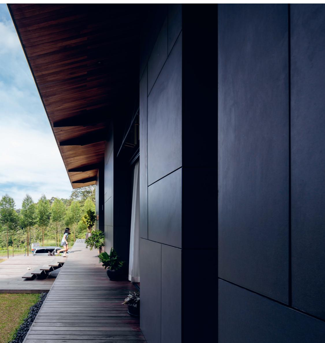
A concealed fixing system was used to hang the fibre cement panels on a metal substructure so that the fixings are not visible. This is a useful method as it creates an even, uninterrupted facade which, not unimportantly, reflects the high quality of the planning.
