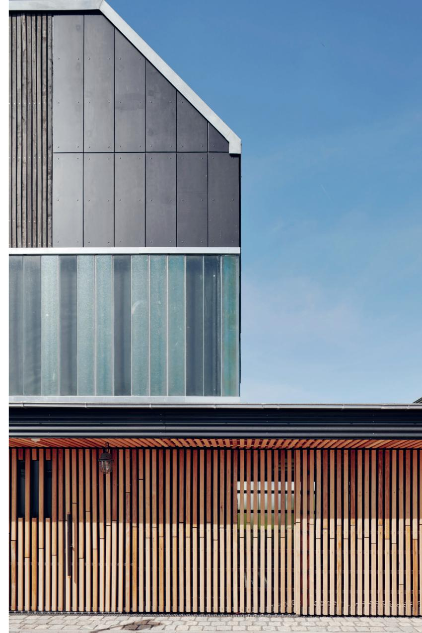
Like all the other elements of the facade the fibre cement panels were renovated before they were reused. Originally green, the panels were made black to create a contrast to the light-coloured wooden elements and the bluish profiled glass. The result is a successful interplay between elongated, standing glass blocks, wood, and glass.
