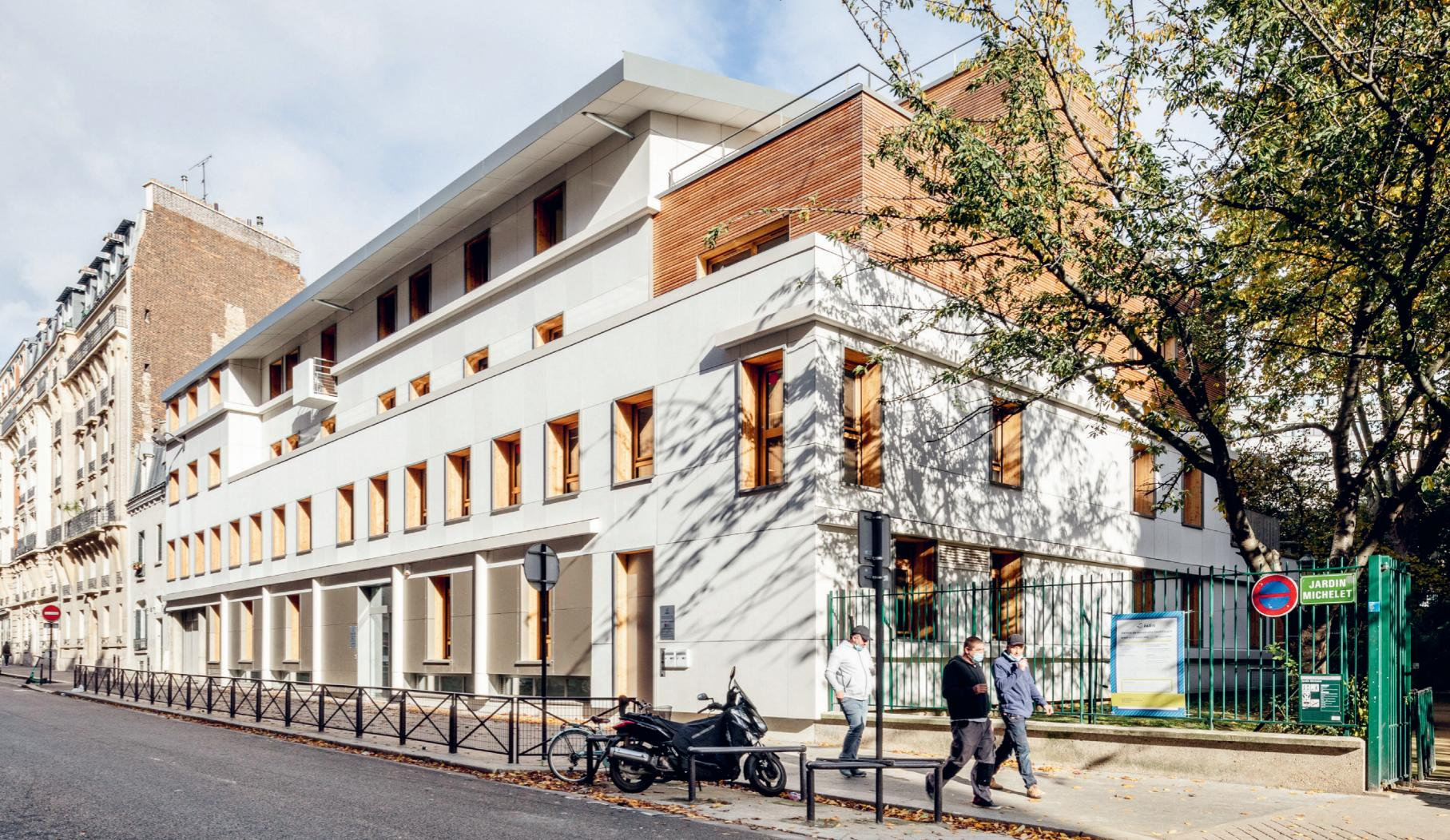
The fibre cement panels meet the sides of the projecting metal window surrounds precisely. They were adapted to the original window sizes and fit perfectly into the grid. The eight-millimetre-wide joints are backed by black strips so that the substructure is invisible.
