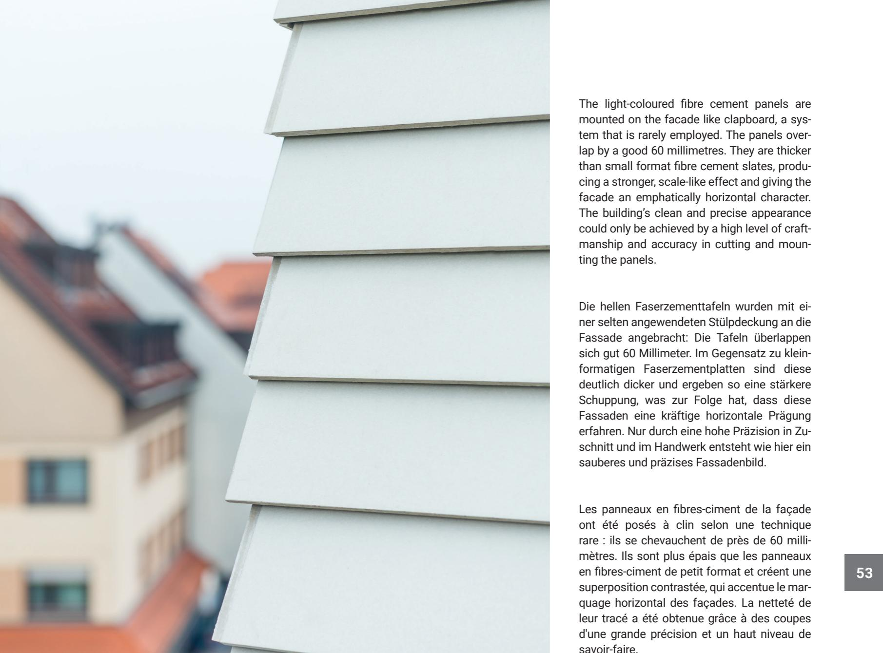
The light-coloured fibre cement panels are mounted on the facade like clapboard, a system that is rarely employed. The panels overlap by a good 60 millimetres. They are thicker than small format fibre cement slates, producing a stronger, scale-like effect and giving the facade an emphatically horizontal character. The building's clean and precise appearance could only be achieved by a high level of craftsmanship and accuracy in cutting and mounting the panels.
