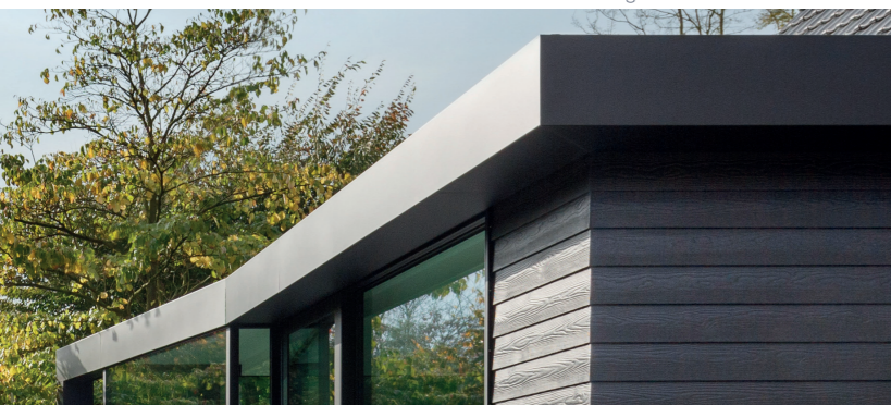
Afwerking dakoversteek in Cedral Board
