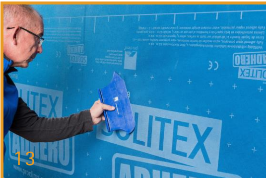
13 Adhere the Entire Section Smooth the membrane into place using PRESSFIX XL adhering the membrane to the substrate, avoiding air bubbles and folds. Apply pressure for good adhesion.
