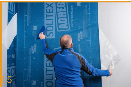
15 Alternative: Vertical Application Attach ADHERO at the highest point. Gradually remove the release film strips by pulling them downward. Apply pressure using PRESSFIX XL.
