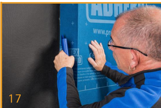
17 Stick Membrane to Reveal Once ADHERO has been cut out, fold it onto the reveal and adhere it in place. Smooth the membrane firmly into place using PRESSFIX XL.
