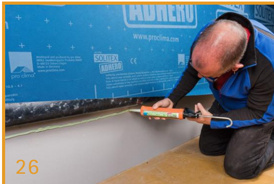
Connect to Foundation When sealing to rough substrates like concrete, apply a bead of ORCON® CLASSIC at a thickness of at least 5 mm. Do not press the adhesive completely flat.
