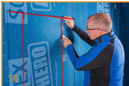
16 Cut Out Window Openings The membrane is first adhered over any window openings. To cut out the opening, cut the membranes as indicated with the red line using a cutter.
