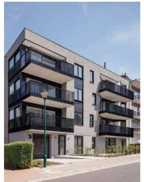
unala- Urban Nation Architects, Wemmel, Belgium
