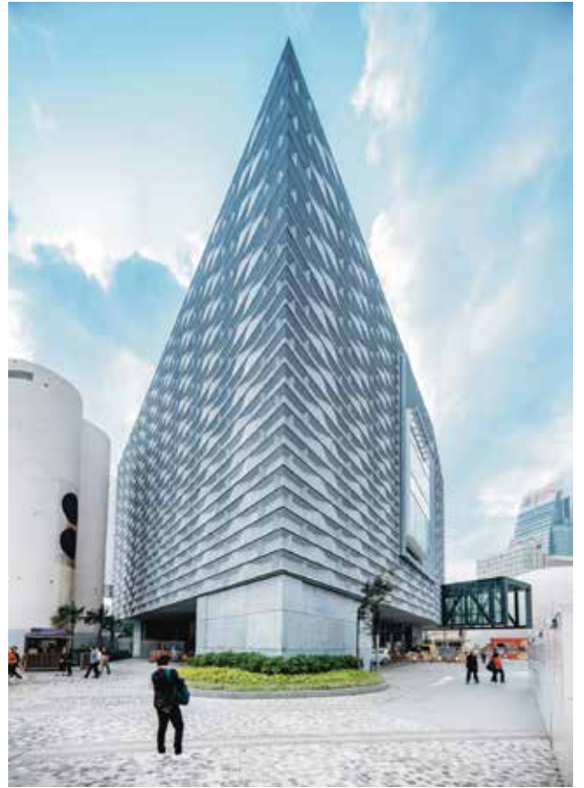
Architectural Services Department, Hong Kong SAR Government, Hong Kong, China
