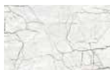
FCS 547 Cracked marble
