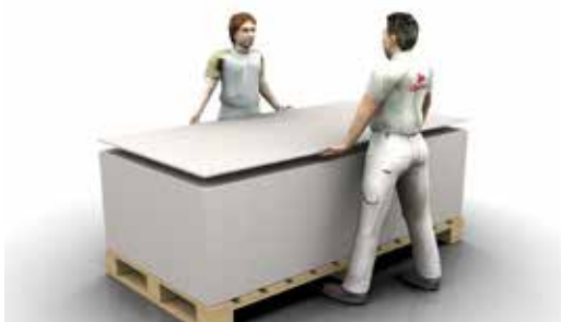
Figure 2 Whenever possible, lift the board from the stack below rather than slide board or drag off the stack. This will prevent damage by scratches to the lower board.
