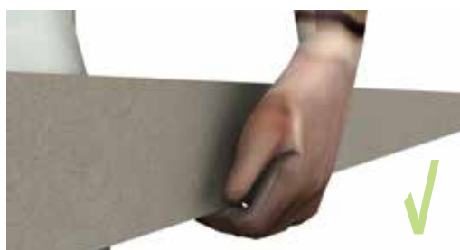
Figure 5 Hold the Kalsi cavity batten vertically at the edge.
