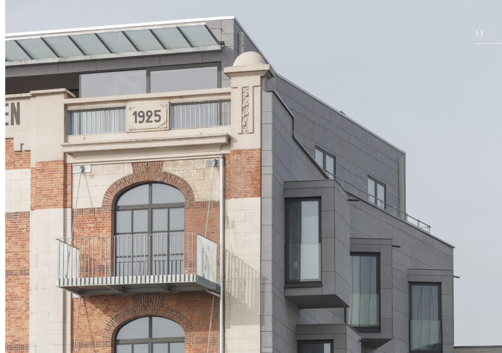
Peynsaert Architecten Aalst, Belgium | EQUITONE [tectiva]®
