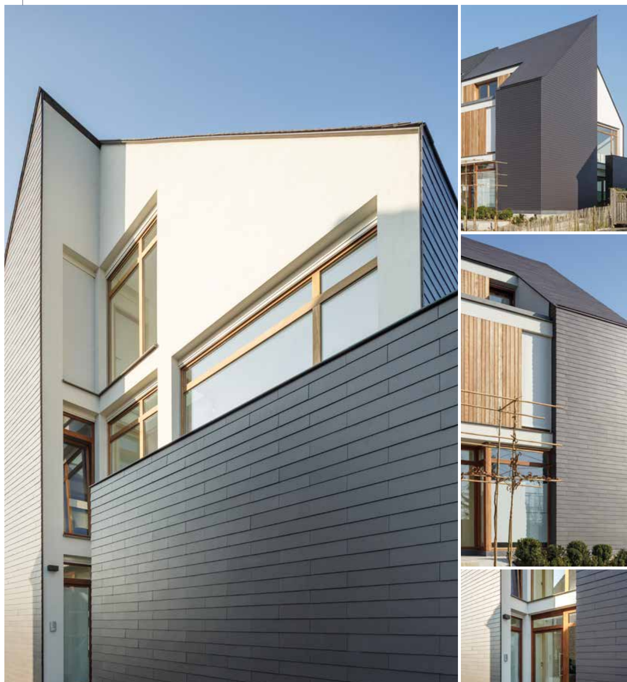
Temse - Architect Bas Wauman (Tielrode)
