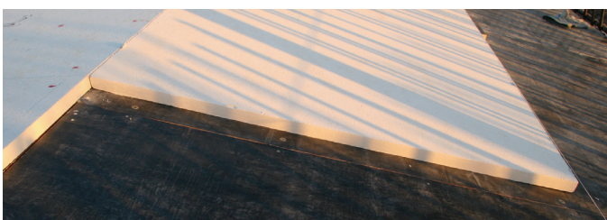
Figure 5: pre-marked screw locations on the boards
