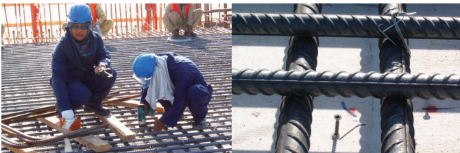
Figure 7: screw insertion
