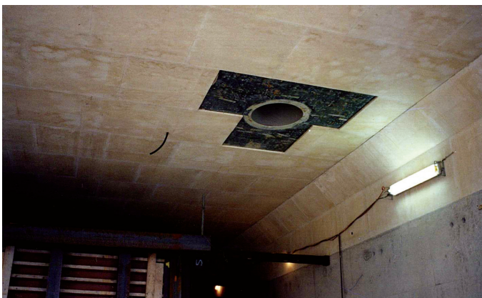
Figure 12: opening of manholes
