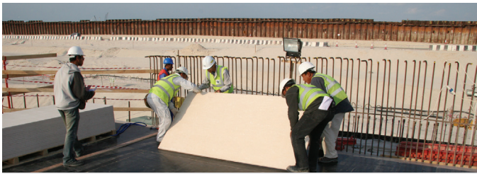
Figure 1: boards laid with the smooth face down using lost formwork
