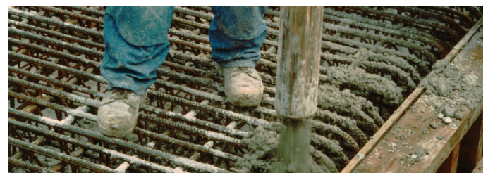
Figure 10: the pouring of concrete
