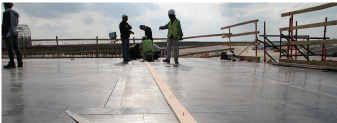
Figure 2: fixed strip of plywood serves as a datum for the first row of boards
