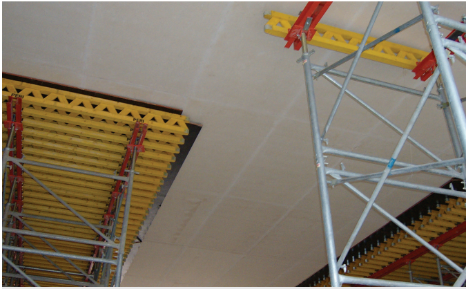
Figure 11: extracted formwork
