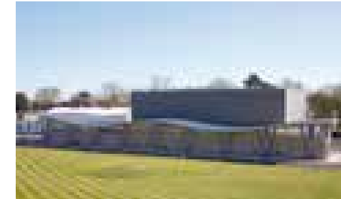
Architects Rivington Street Studio, London, United Kingdom Project Manager Artelia, London, UK Location St. Mary's University College, Waldegrave Road, Twickenham, Greater London, UK Photos Marley Eternit (left, right top), Simon Kennedy (right bottom)
