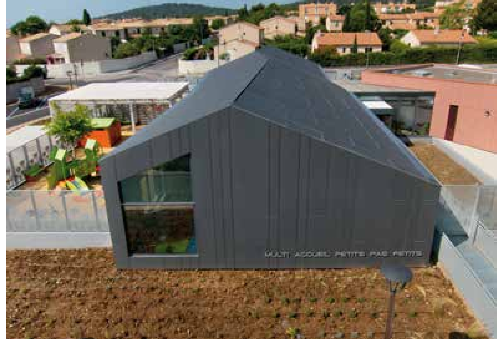
Above: All exterior walls as well as the double-pitch roof are clad with fibre cement panels.
