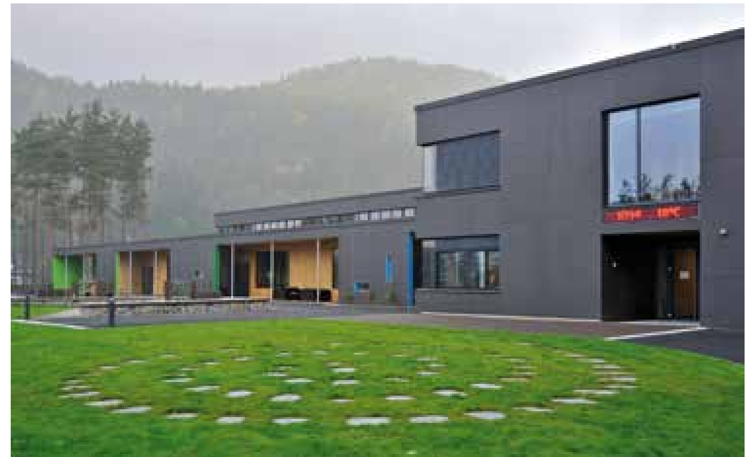
South elevation, the refurbished building on the right, boasting a new fibre cement façade; the new building to the left
