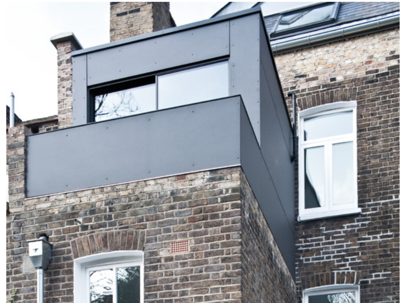
Fibre cement panel cladding on the extension in contrast to existing brick masonry.
